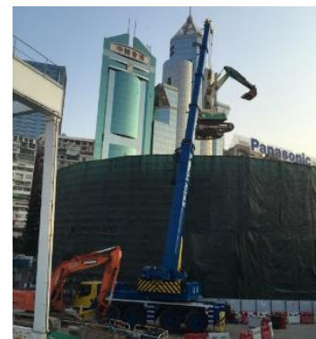
Lifting 20t Machine by a 100 Ton Crane to Roof 用 100 噸大吊機吊運 20 噸拆卸機械上樓頂
